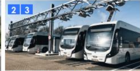
Electric bus charging station
